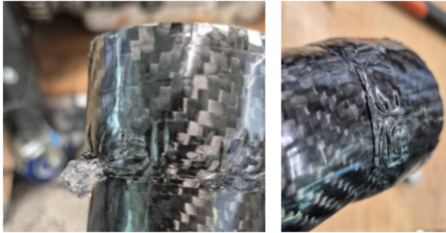
Figure 51: visual inspection of test Article 2, (left) pooling of epoxy and heat shrink tape. (right) rippling caused by overheating of heat shrink tape
